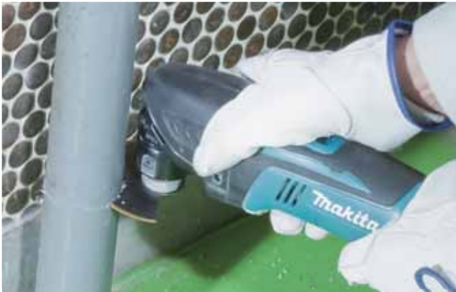
Cutting PVC, FRP pipes
