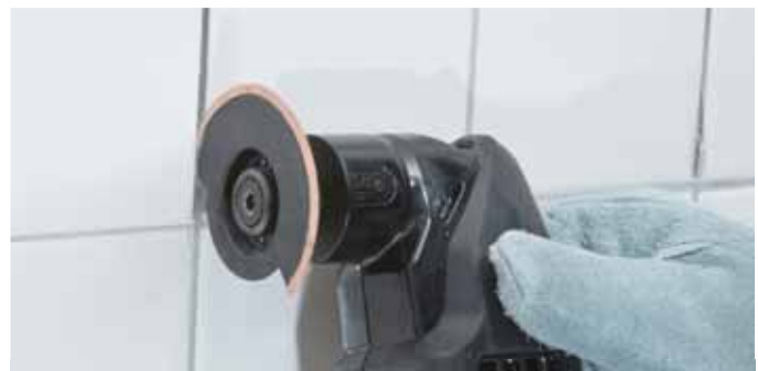
Routing joints on wall tiles
