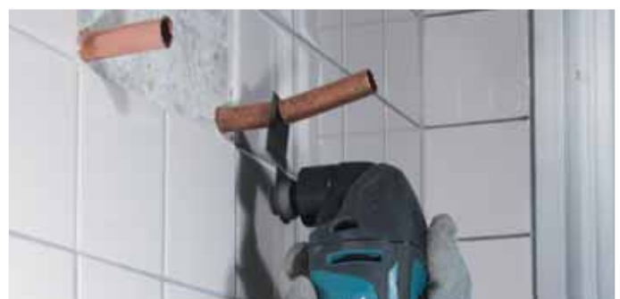
Cutting copper pipe
